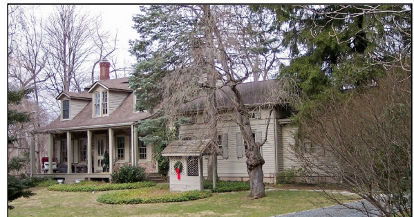
The recent frame wings at the right attached to the David and Cornelius Van Horn House use traditional materials that are compatible with the early stone house. They are set back from the front wall of the historic section.
