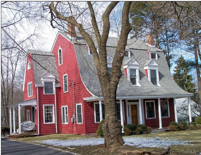
This house may incorporate an earlier structure, but its exterior style is Dutch Colonial Revival with flaring gambrel roofs on both main section and narrow side wing.
