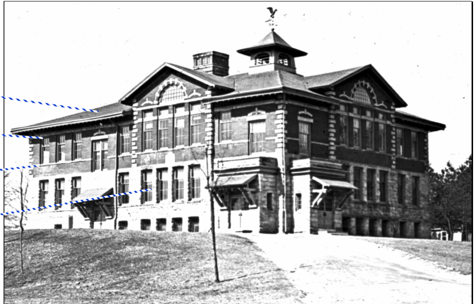
The Village School was initially constructed in 1899-1900 and subsequently received a number of additions. The 1907 addition, shown at the left, and the 1912 addition, built after this photograph was taken, continue the original Renaissance Revival style.
