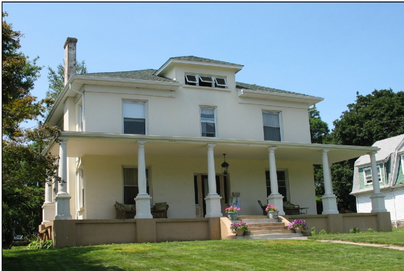
This 3-bay-wide Foursquare is unusual in Closter as it is constructed of poured concrete.
