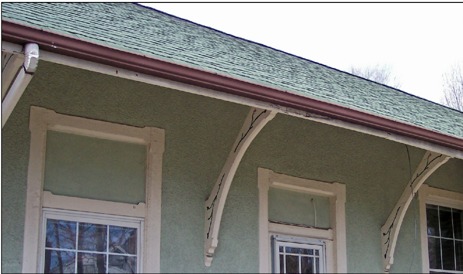
The station building's original braces and overhanging roof remain.
