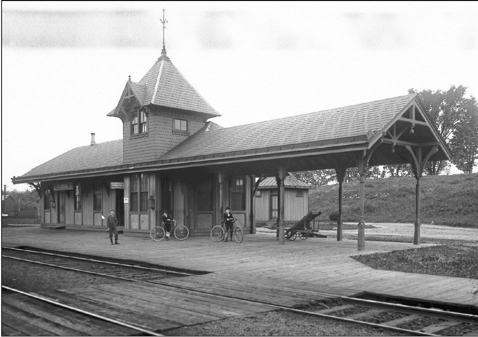
This late 19 th century photograph shows the Stick Style Closter railroad station of 1875 before it was moved and converted into a residence. Note the applied vertical boards suggesting framing, the heavy decorative trusses in the gable, and the braced overhanging roof.
