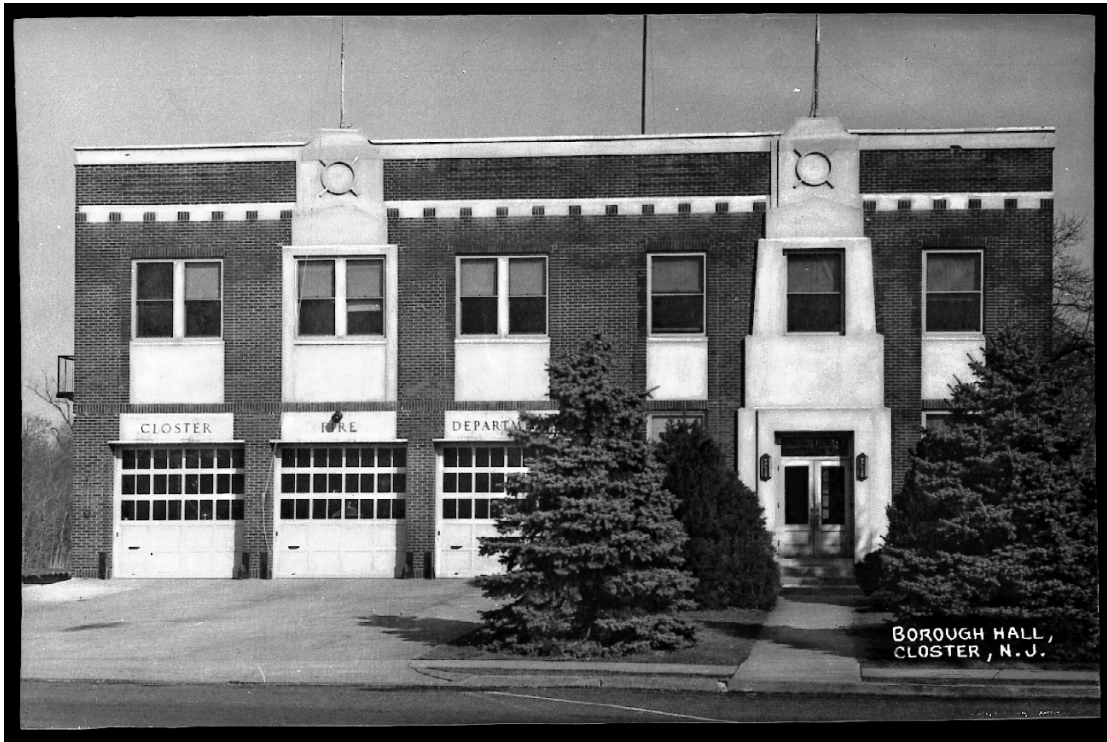
Historic Photo of Closter Borough Hall showing garage doors and projecting flagpoles atop cast stone ornamentation, c. 1940
