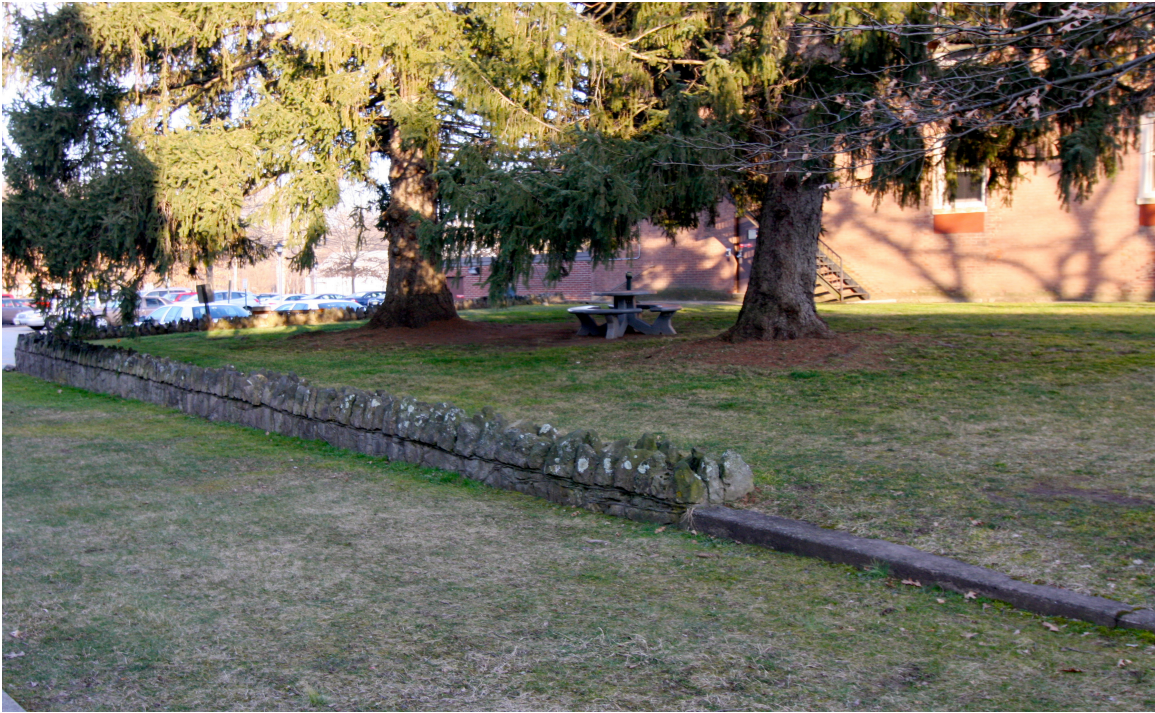
Rubble stone wall at west side of property
