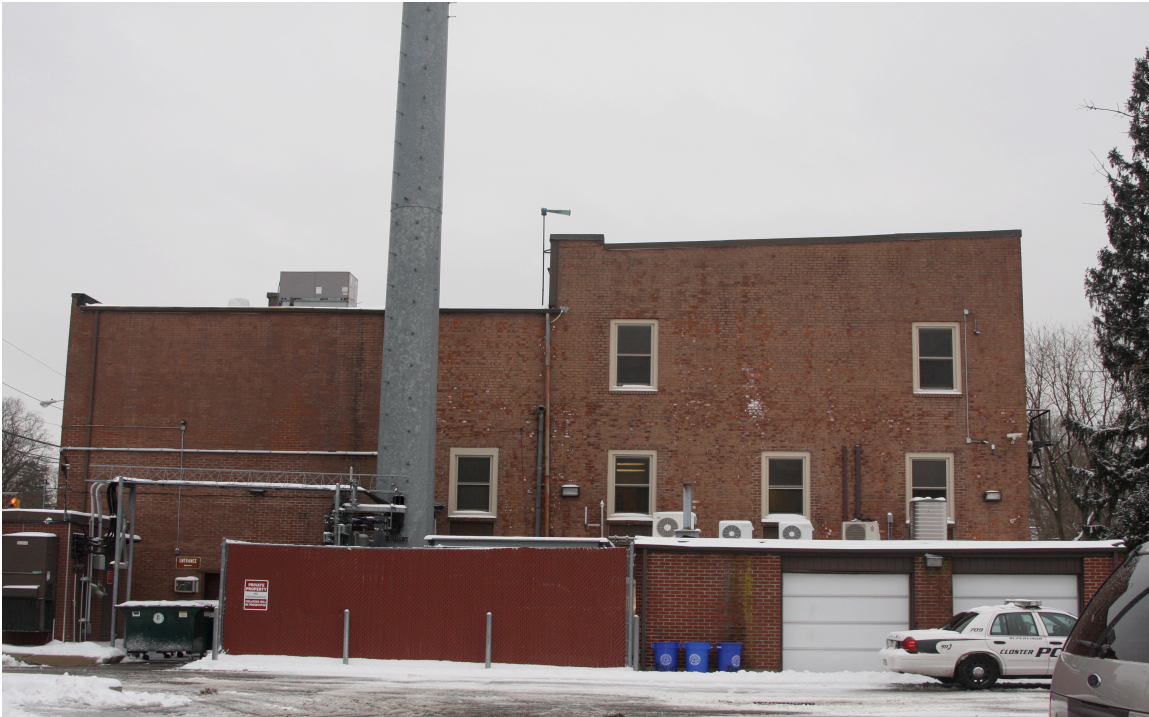
Rear of building showing garage addition and base of cell tower monopole
