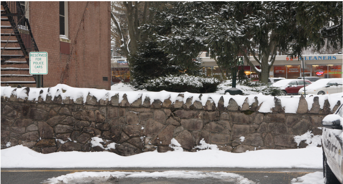
Rubble stone wall at rear of building
